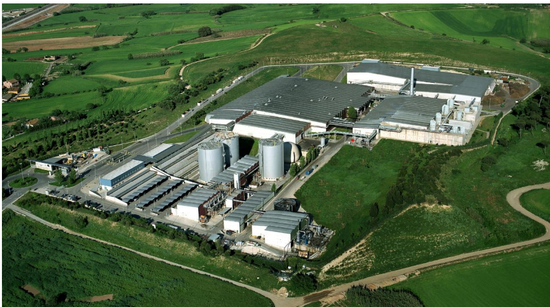
Figure 7: Ecoparc 2 aerial view (image author: Ecoparc 2)
