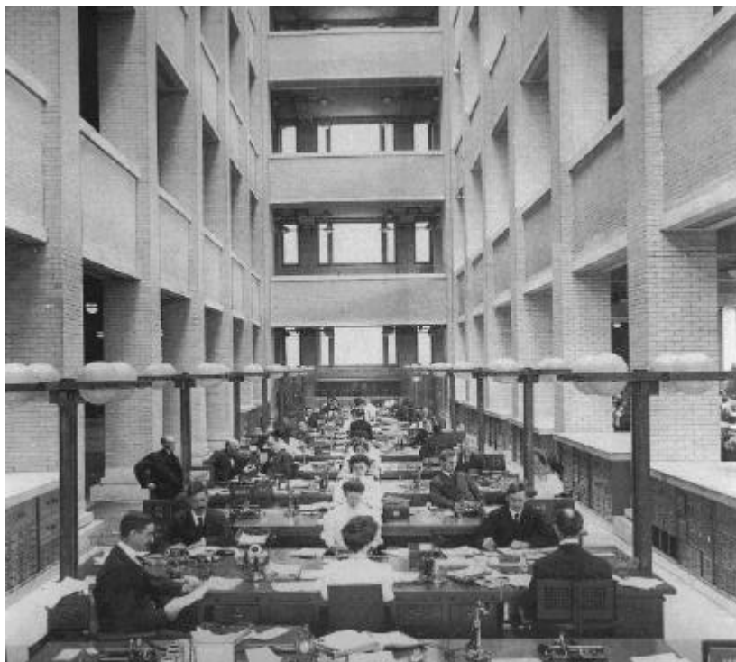
The Larkin Building. Buffalo. New York. 1904
