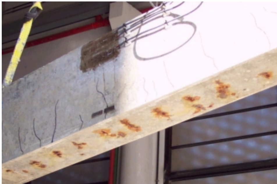
Figure 6.4.17. Corrosion of the shear reinforcement after 12-months of chlorides attack.
