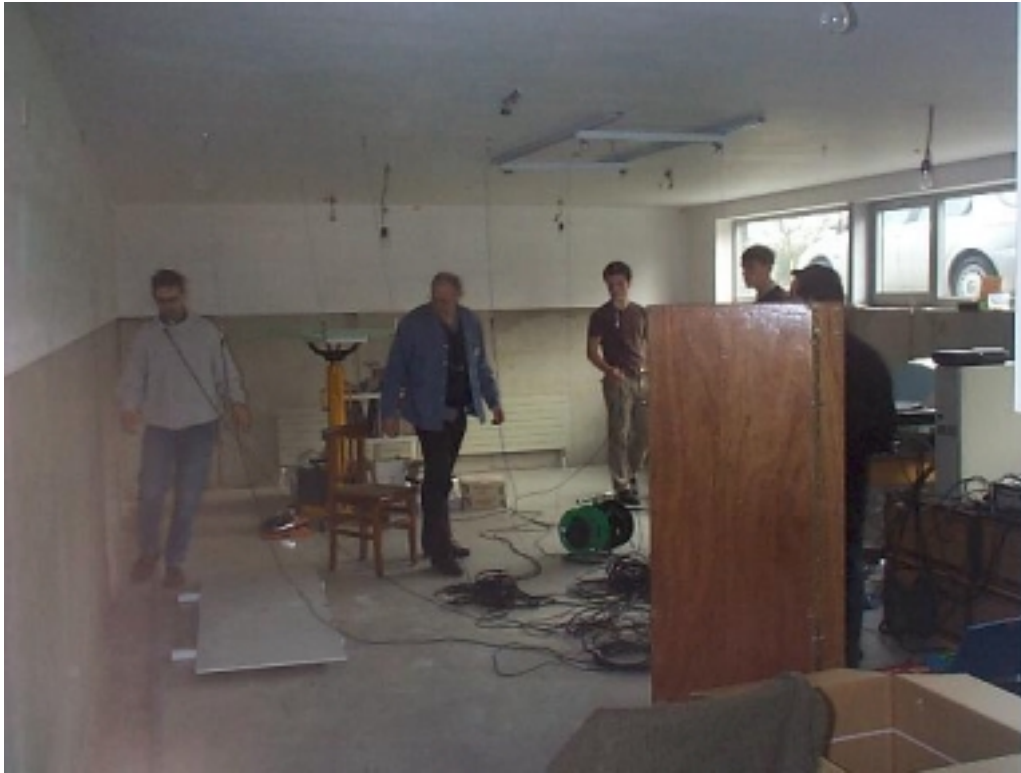
Figure 7.4. Deployment of dynamic sensors in the slab
