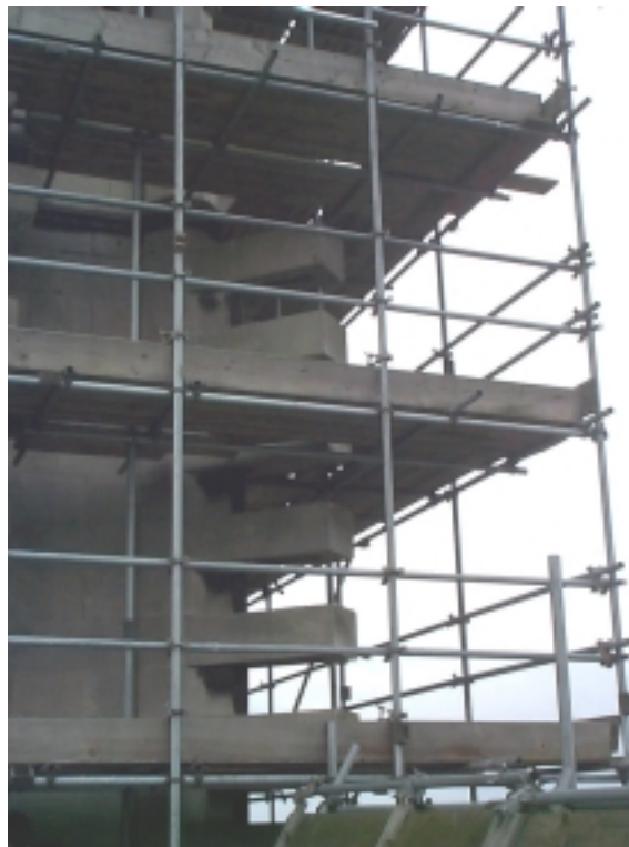
Figure 7.45. Frameworks deployed to avoid stone falling (right).
