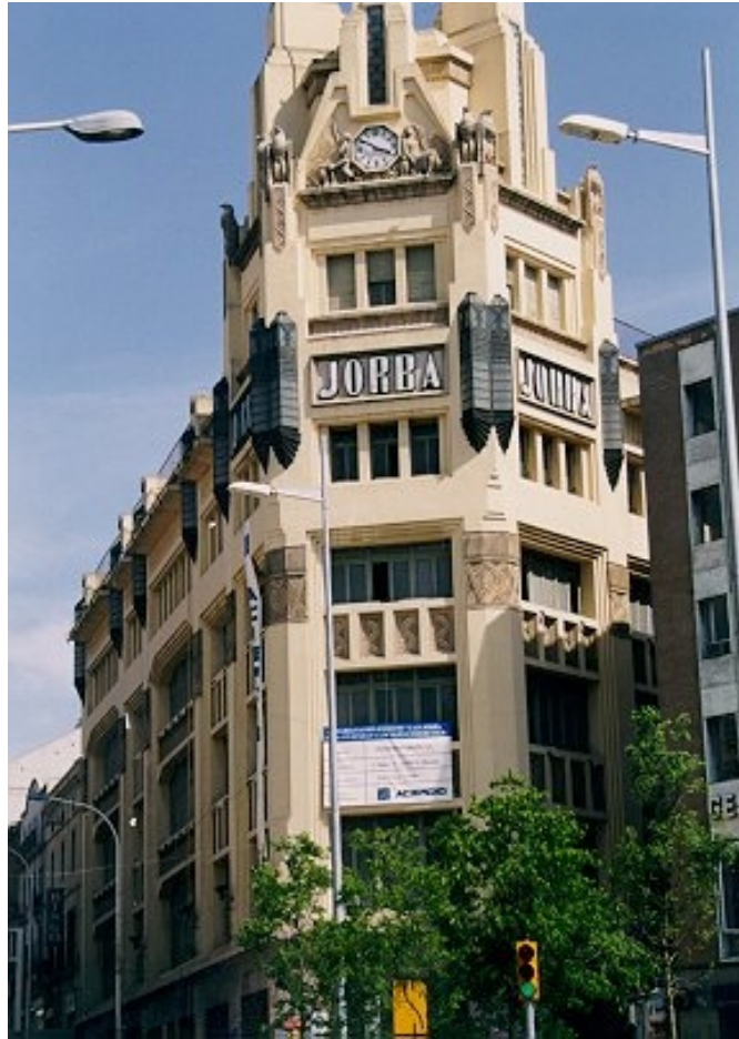
Figure 7.14. Main façade of the studied building.
