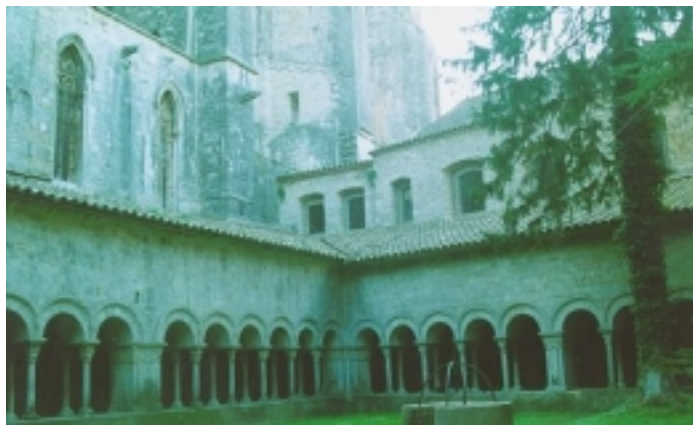
Figure 7.26. Cloister view with the Cathedral behind.
