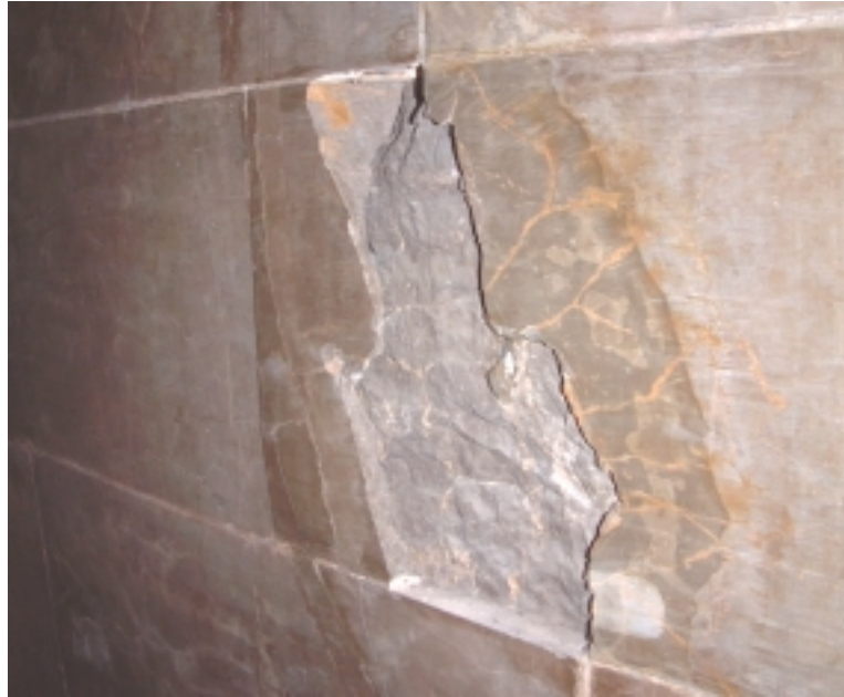
Figure 7.37. The “exploded” stone.
