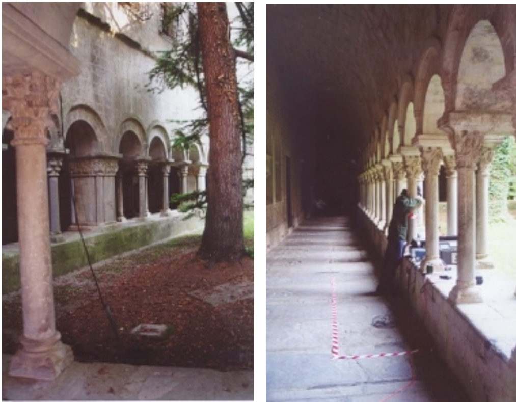
Figure 7.24. General views of the cloister and tested columns.
