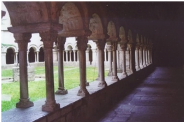
Figure 7.23. General view of the cloister and tested columns.
