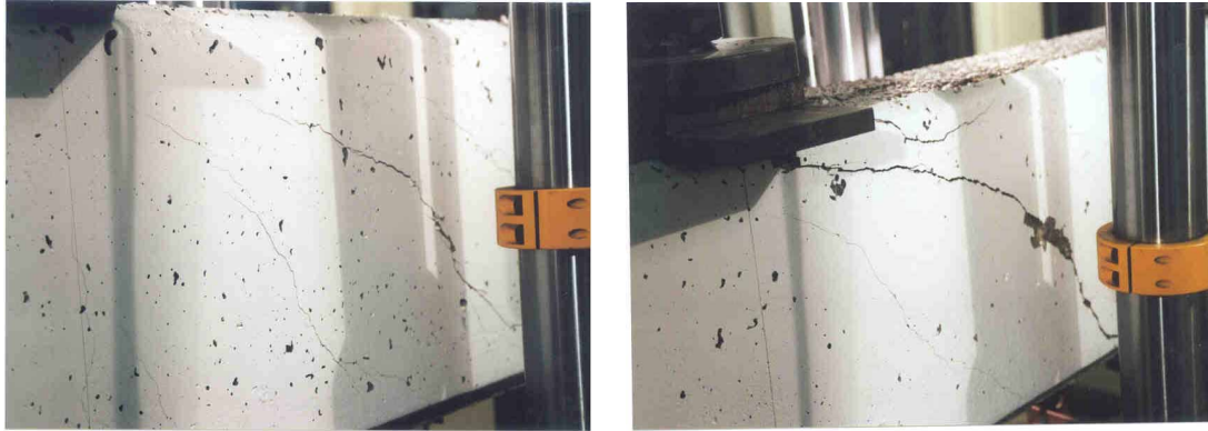
Figure 4.1: Cracking prior to failure and at failure in a beam with web reinforcement. Concrete spalling near the diagonal crack.
