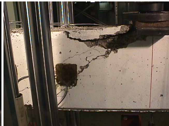
Detail of the compression flange at failure
