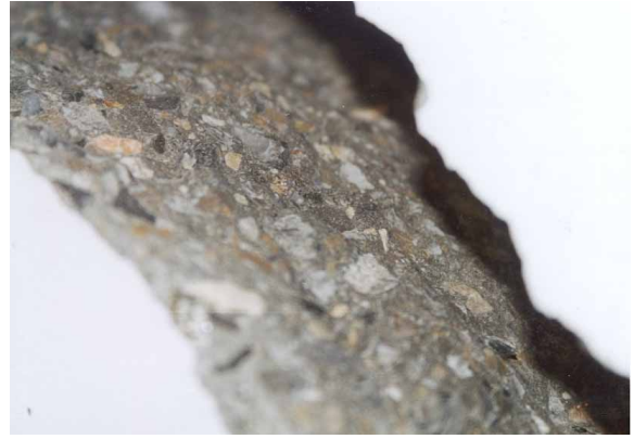
Crack surface at failure
