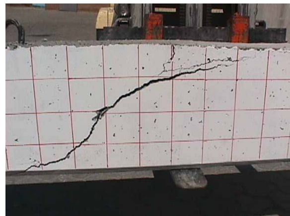
Cracking at failure ( V = 108.14 \text{ KN} )
