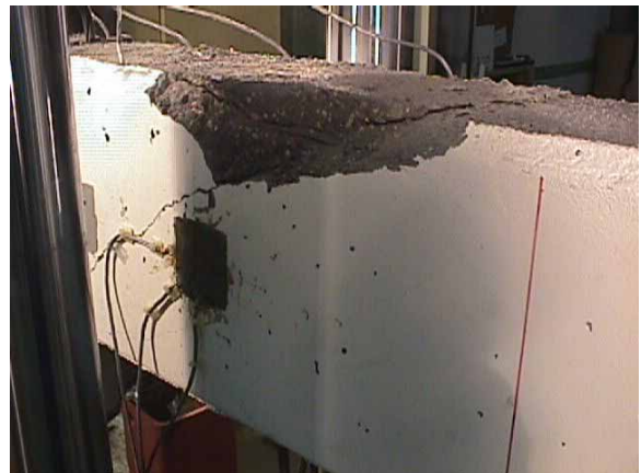
Detail of the compression flange at failure
