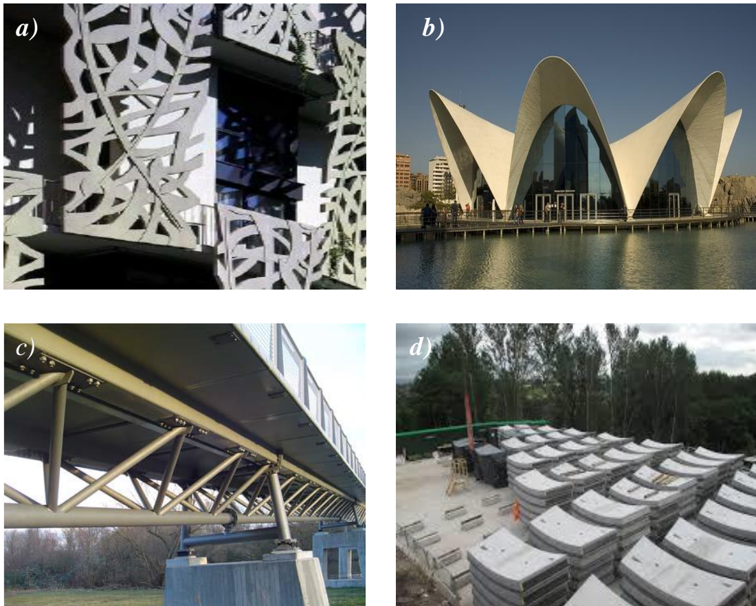
Figure 1.1 – Field applications of HPFRCCs: a) façades panels, b) shell roof, c) high performance deck glued to a 3-D steel truss and d) precast elements.
