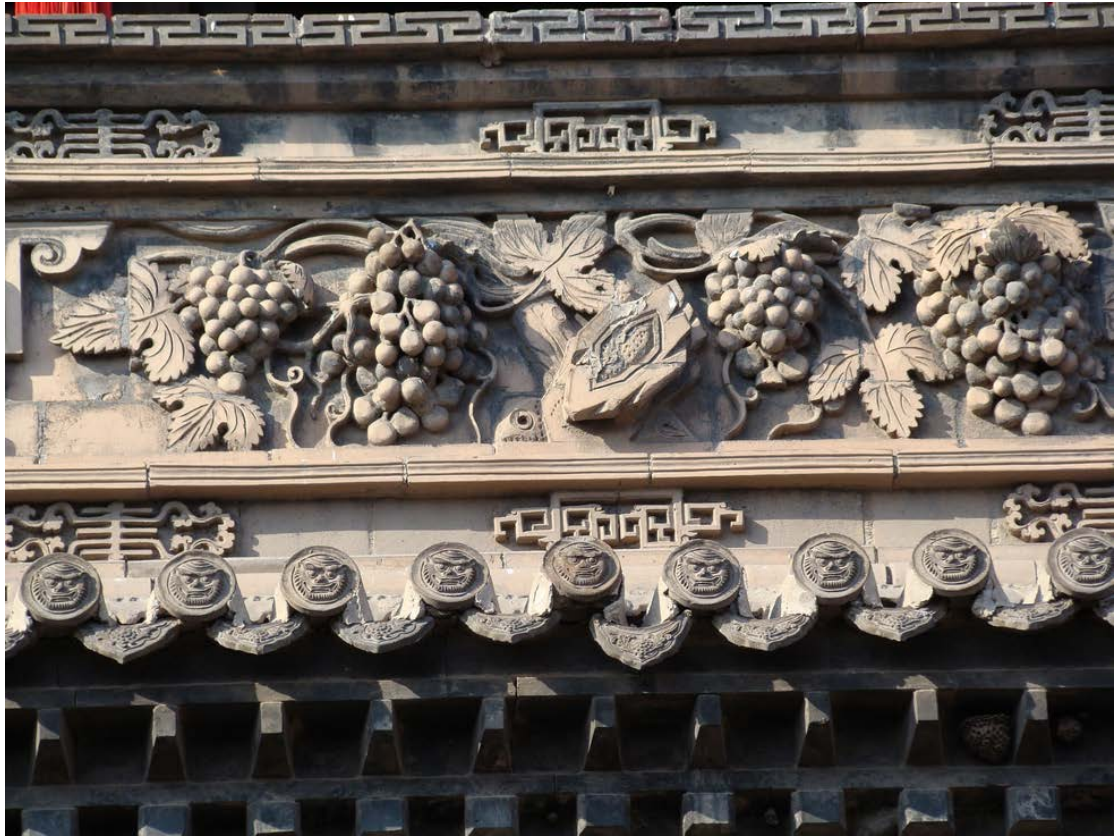
Figure 3-33 Brick carving of Qiao's Courtyard, Shanxi Province
