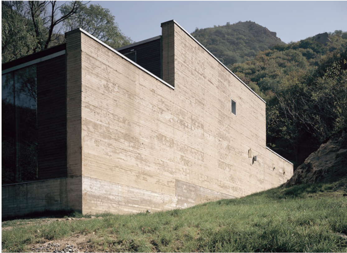
Figure 4-22 Rammed earth wall of the Split House
