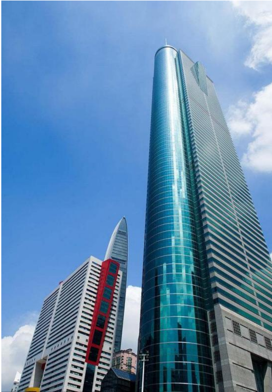
Figure 4-73 Diwang Building, Shenzhen
