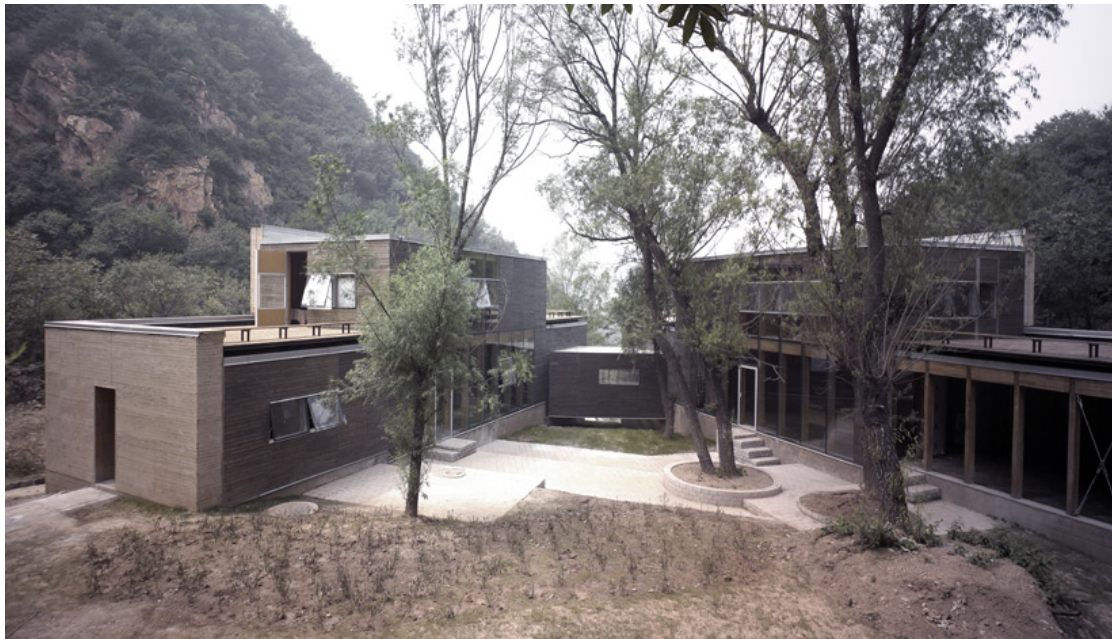
Figure 4-20 Courtyard of the Split House
