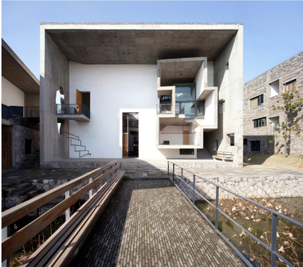
Figure 4-49 A teaching building of Xiangshan Campus, China Academy of Art, Phase 2
