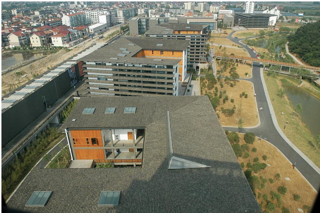
Figure 4-36 Aerial view of the Xiangshan Campus of the China Academy of Art, Phase 1
