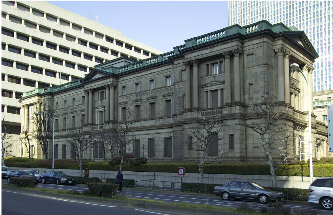
Figure 5-29 Bank of Japan Headquarters
