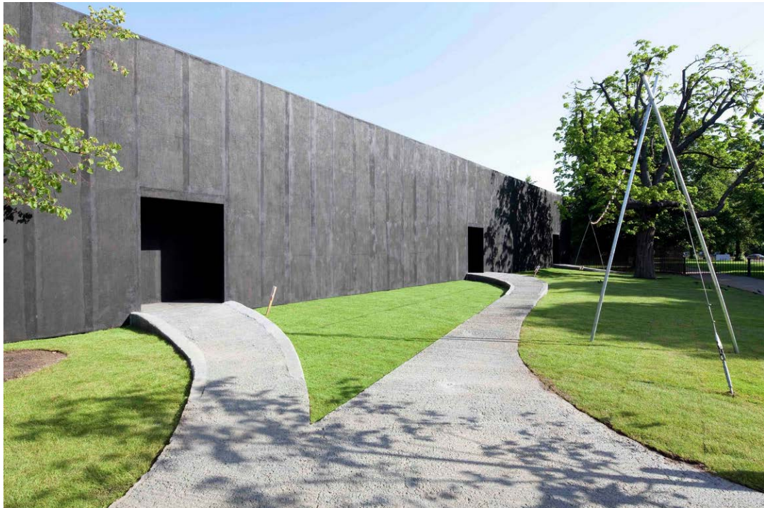
Figure 5-24 Facade of the 2011 temporary Serpentine Gallery pavilion
