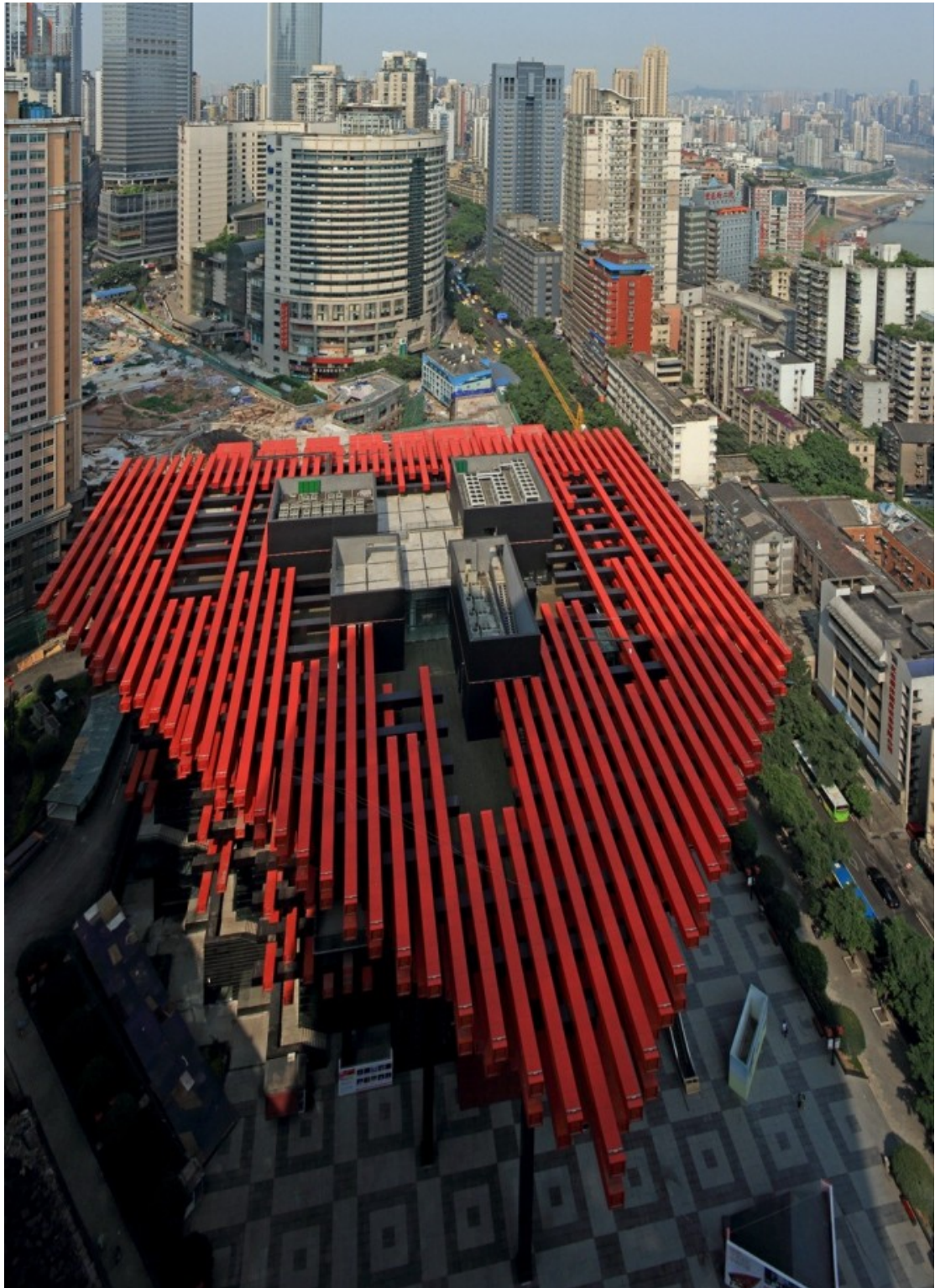
Figure 6-13 Aerial view of Chongqing Guotai Arts Center
