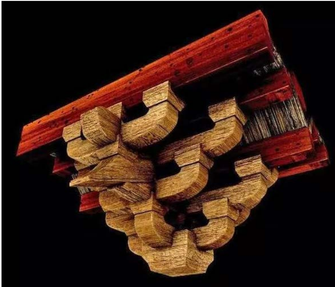
Figure 4-29 Traditional Dougong timber element
