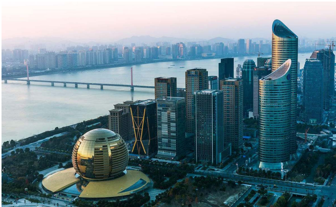
Figure 4-7 Hangzhou Qianjiang New City
