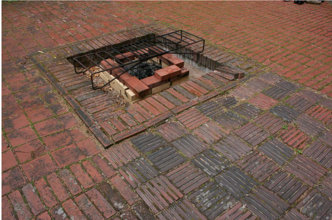
Figure 5-4 Muuratsalo Experimental House's fireplace
