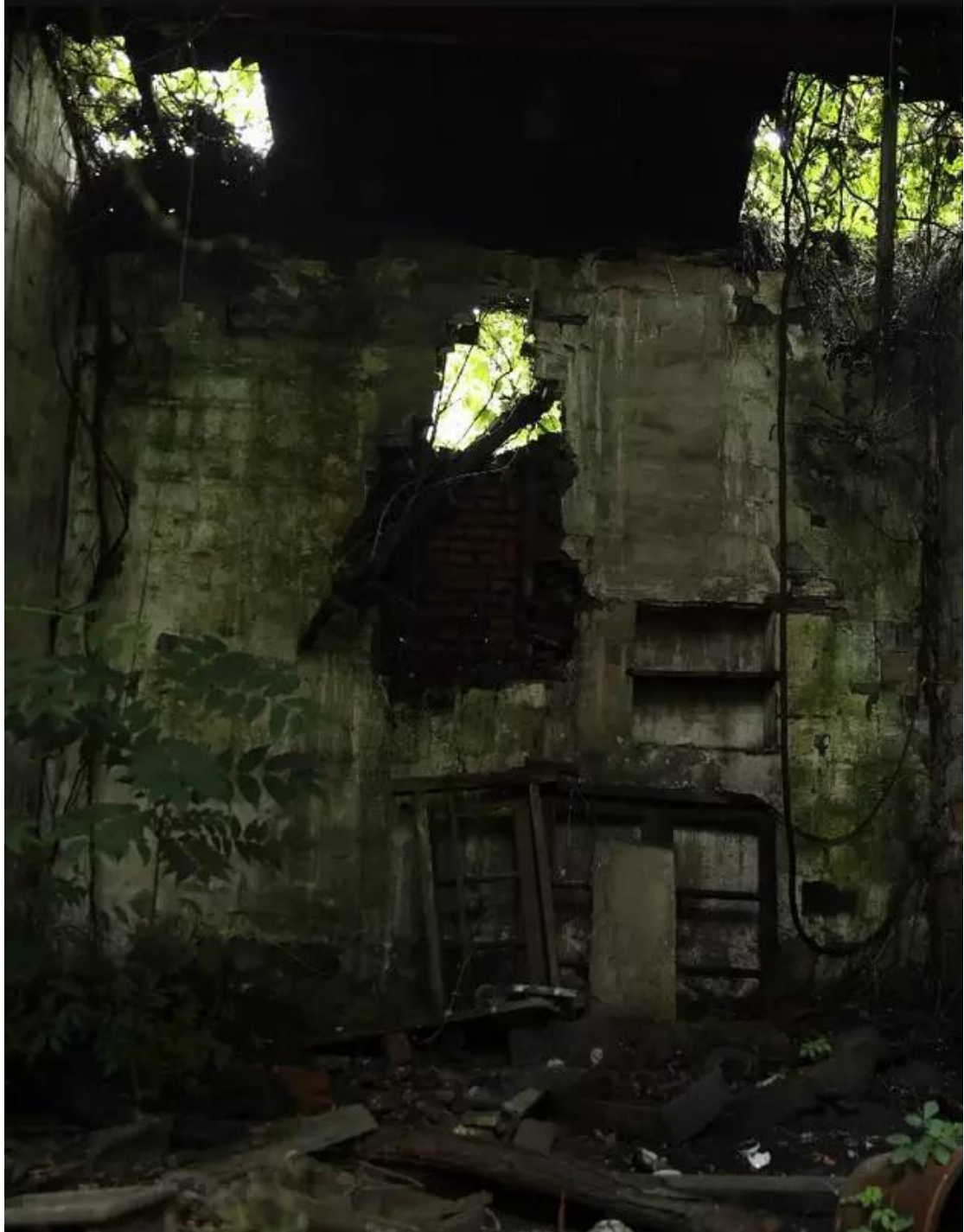
Figure 4-82 Wang family's ancestral home before its rebuilding
