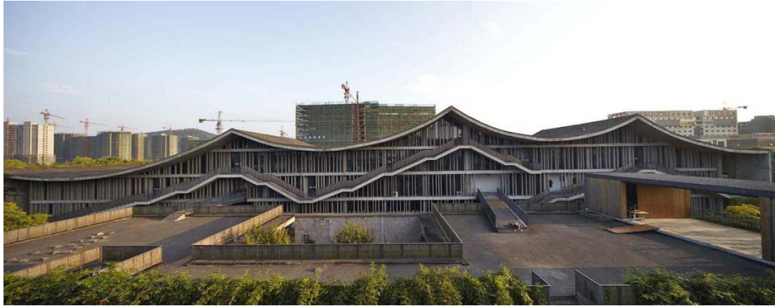
Figure 4-44 Building No. 19 of Xiangshan Campus, China Academy of Art, Phase 2
