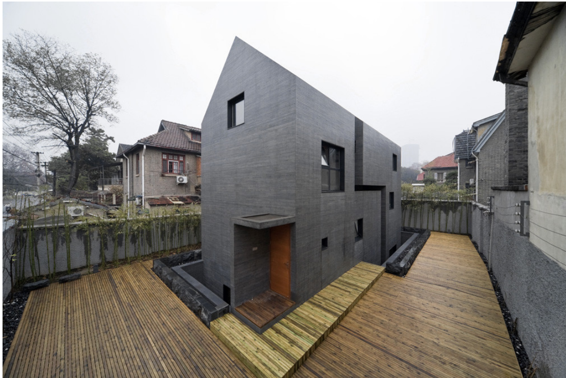
Figure 6-15 Concrete Slit House
