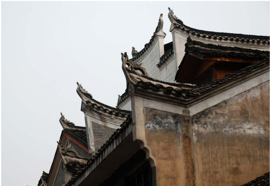
Figure 3-23 Gables in Fenghuang old city
