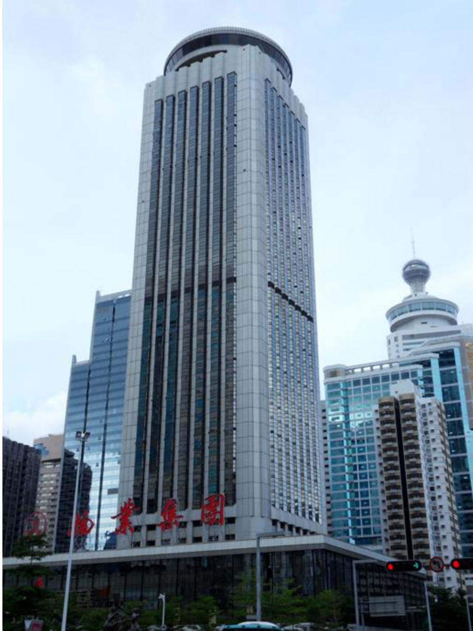
Figure 4-72 International Trade Building, Shenzhen
