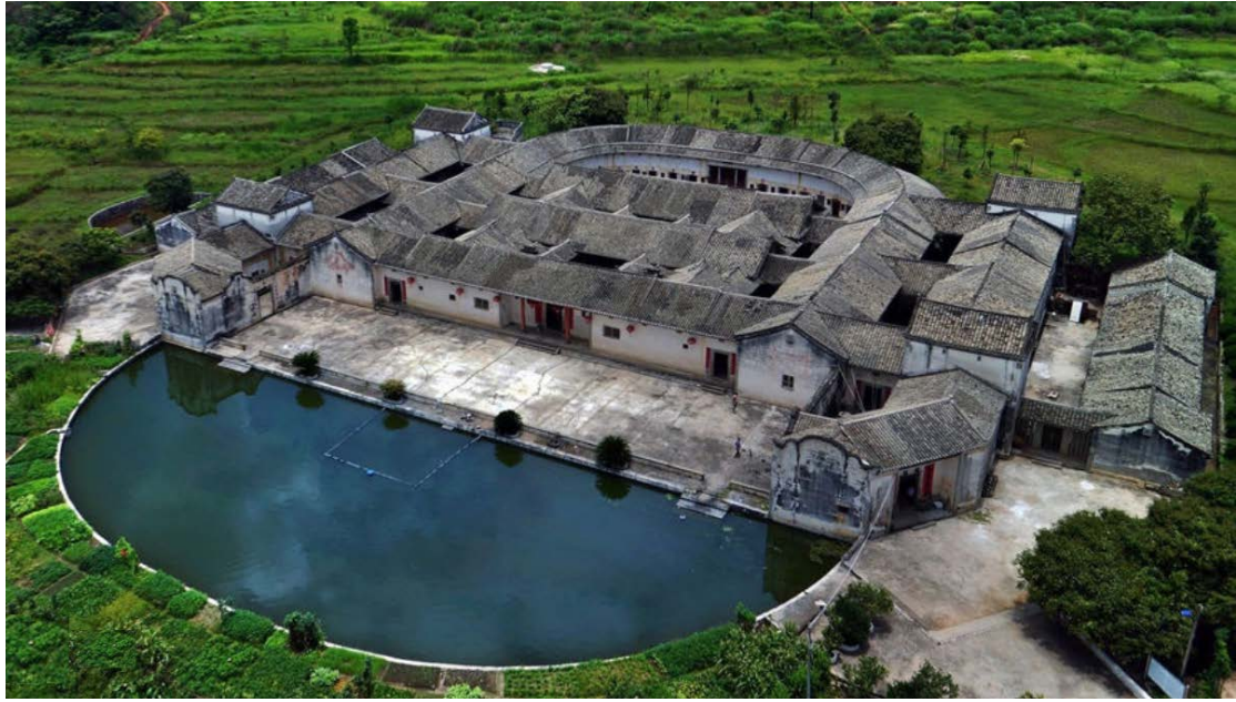
Figure 3-40 Pan'an house, Xingning, Guangdong
