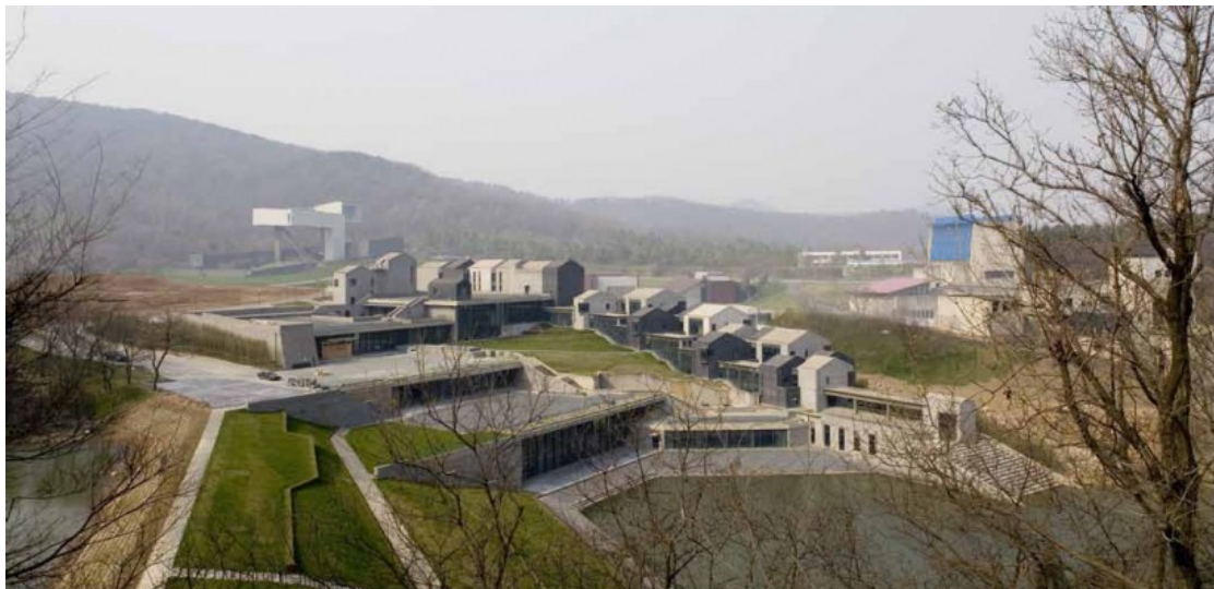
Figure 6-19 Aerial view of Reception and Dining Center of CIPEA
