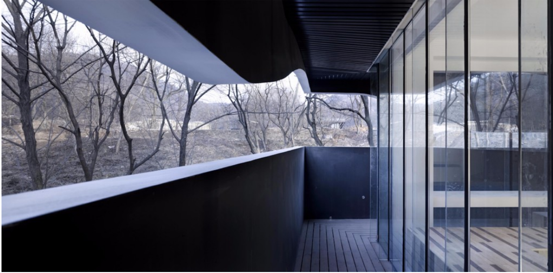
Figure 6-26 the corridor of the No.4 house of CIPEA
