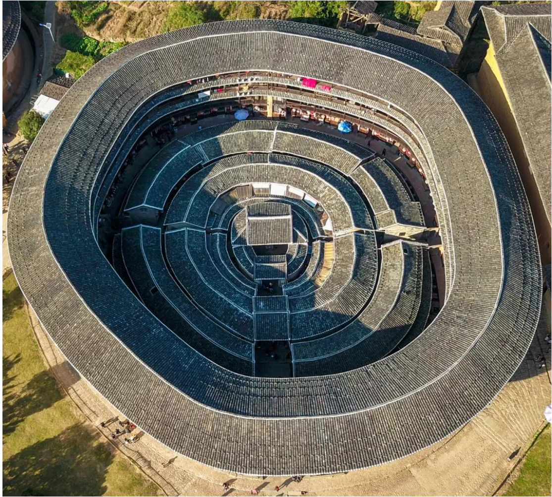
Figure 3-12 Hakka round houses, Longnan, Ganzhou, Jiangxi Province
