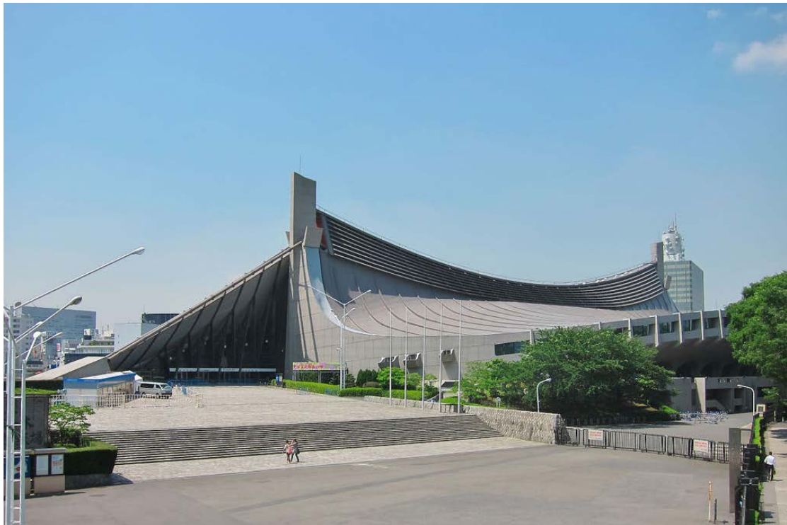
Figure 5-35 Yoyogi National Gymnasium
