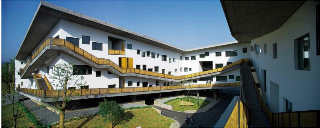
Figure 4-46 Building No. 18 of Xiangshan Campus, China Academy of Art, Phase 2
