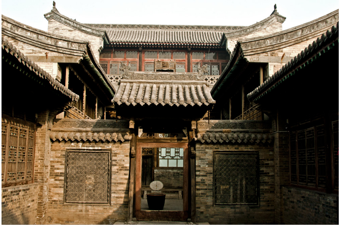
Figure 3-8 Wang's Courtyard, Lingshi County, Shanxi Province
