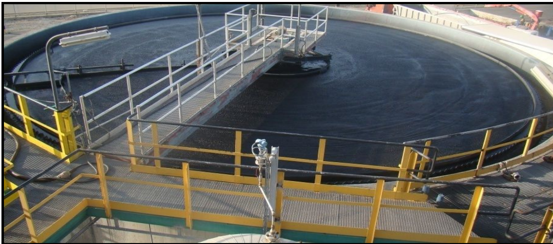
Figure 2.13 Surface of a clarifier belonging to an activated sludge system which experiences a filamentous bulking
