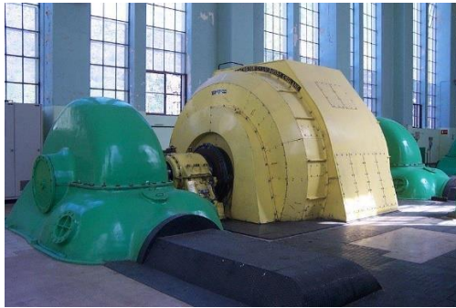
Figure 2.4. Views of the Pelton unit
