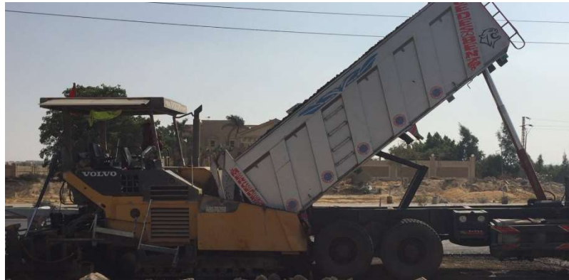
Figure 4- 10: Paving finisher
