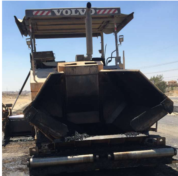
Figure 4- 13: Paving finisher waiting the asphalt trucks
