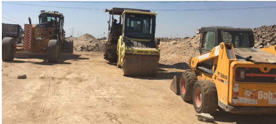
Figure 4- 12: Waiting for inspecting the finished activity
