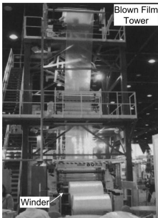
Figure 1-13 Macchi blown film tower [77].
