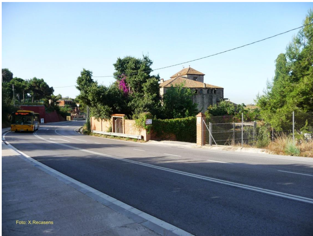
Figure 4 BDN cellar. Photo: X. Recasens
