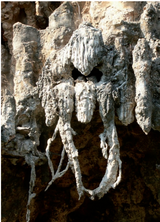
Fig. 3. Giant's head, which serves as a fountain. Detail of the facade of the Cova Cascada (1907).
