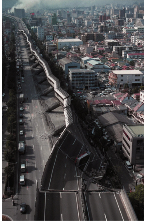
Fig. 1.1: Scene of Kobe, Japan, after the 1995 Hyogo-ken Nanbu earthquake (magnitude 7.2), showing a collapsed section of the Hanshin Express-way. Photography extracted from Pan-Asia Newspaper Alliance.
