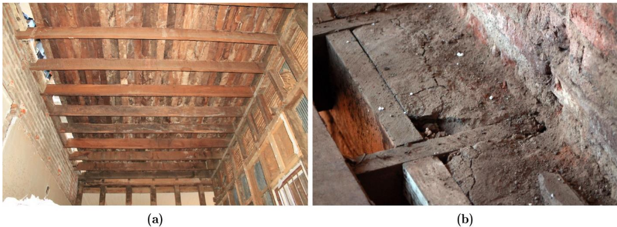
Figure 7-22. Timber-masonry buildings: (a) masonry and timber frame interaction and (b) joist-masonry wall connection.
