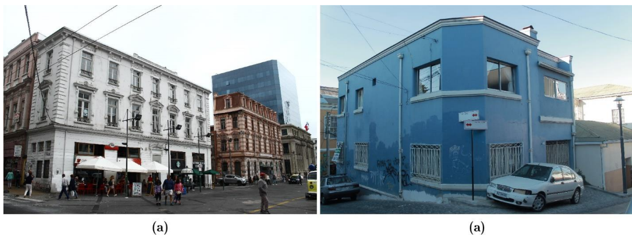
Figure 7-24. Masonry buildings (a) Historical constructions in Sotomayor square (label 99 and 100 in Figure 7-21), and (b) reinforced masonry building with visible damage in masonry (label 40).
