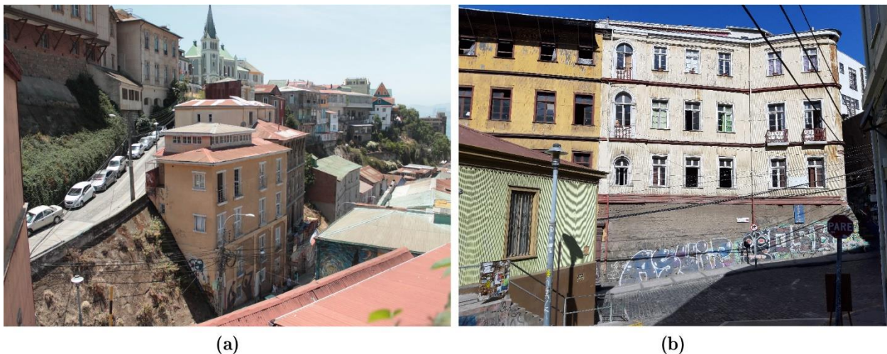
Figure 3-20 (a) Buildings adapted to the stepped hillside in the Almirante Montt street, and (b) a mixed stone and masonry basement in the Urriola street.
