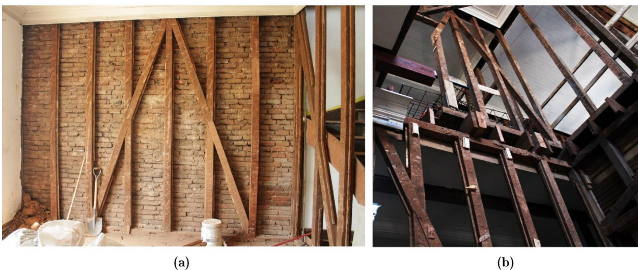
Figure 3-23. Timber frame load bearing systems: (a) bare frame wall built next to a masonry sidewall, and (b) platform frame configuration (Jiménez 2015).
