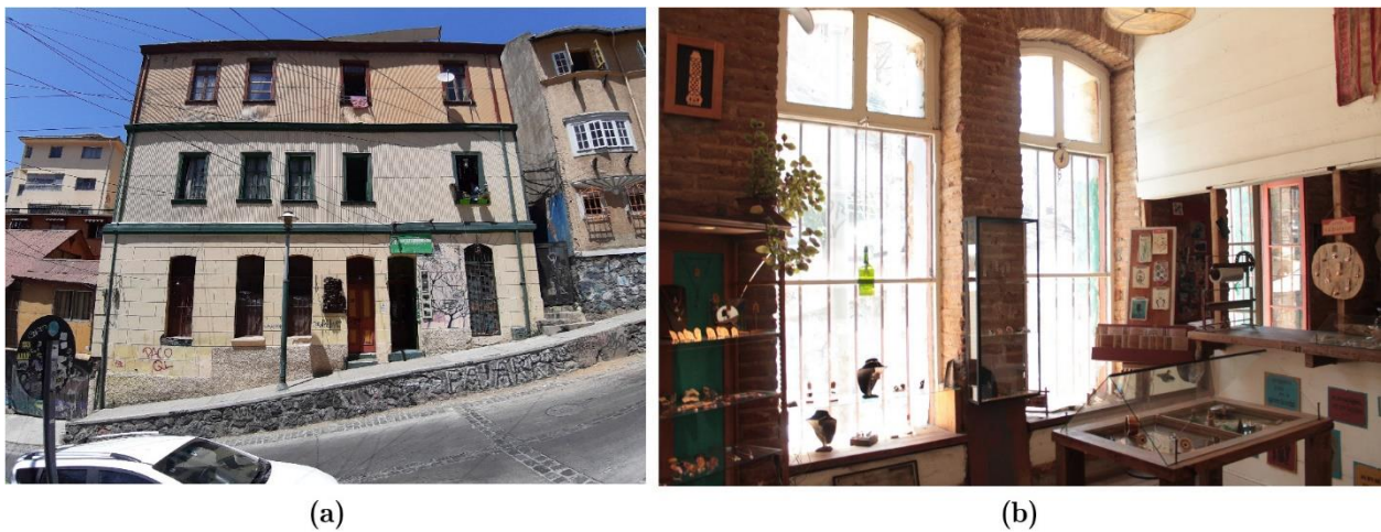
Figure 3-22. Hybrid timber-masonry building with masonry walls at the ground floor and timber frames at upper levels: (a) façade, and (b) internal view of the brick masonry wall.
