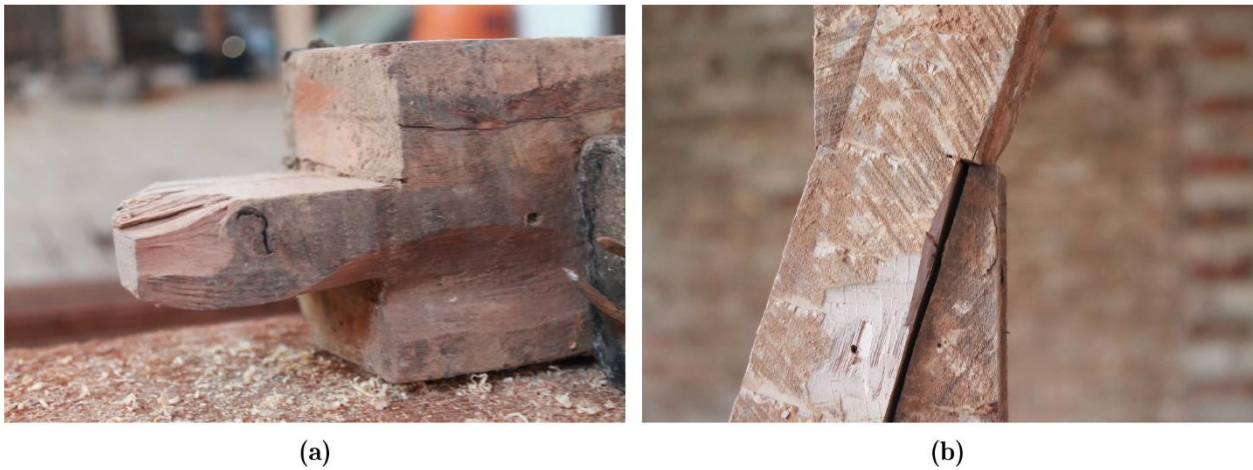
Figure 3-24. Carpentry joints in timber frames: (a) tenon at the end of a stud, configuring the mortise-and-tenon joints, and (b) stud and diagonal connected by a notched joint (Jiménez 2015).
