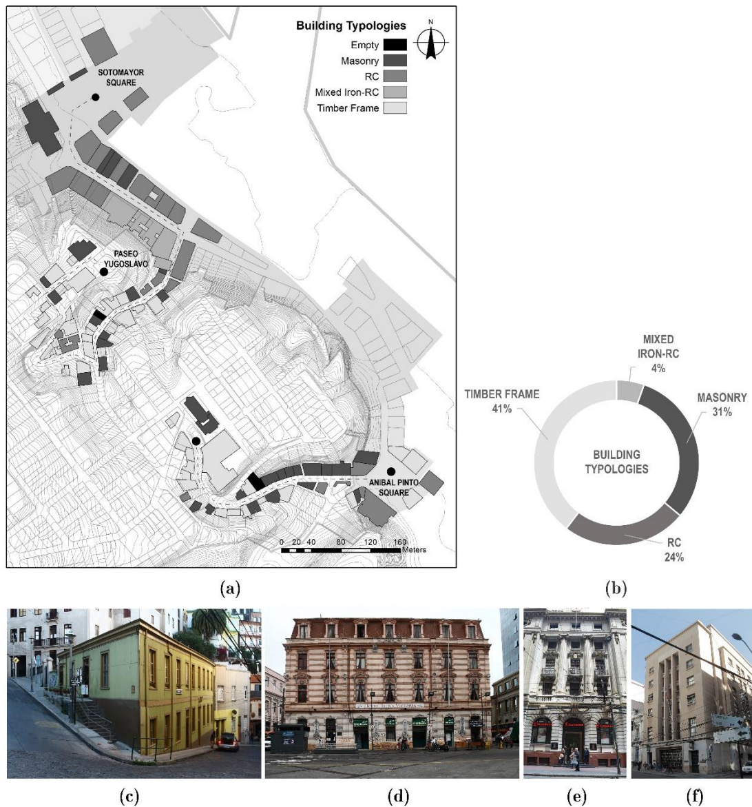
Figure 4-24. GIS mapping of the structural typologies (a) and their statistical distribution (b). Representative timber frame dwelling (c), masonry building (d), mixed iron-RC building (e) and RC building (f).
