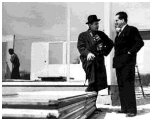
Figura 44. The Packaged House System para General Panel Corporation Walter Gropius y Konrad Wachsmann.
