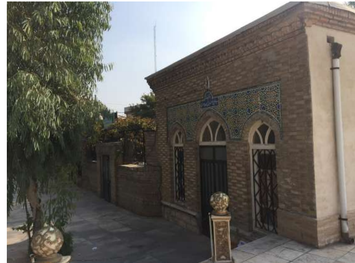
Fig.96: Modern brick building, 2020
