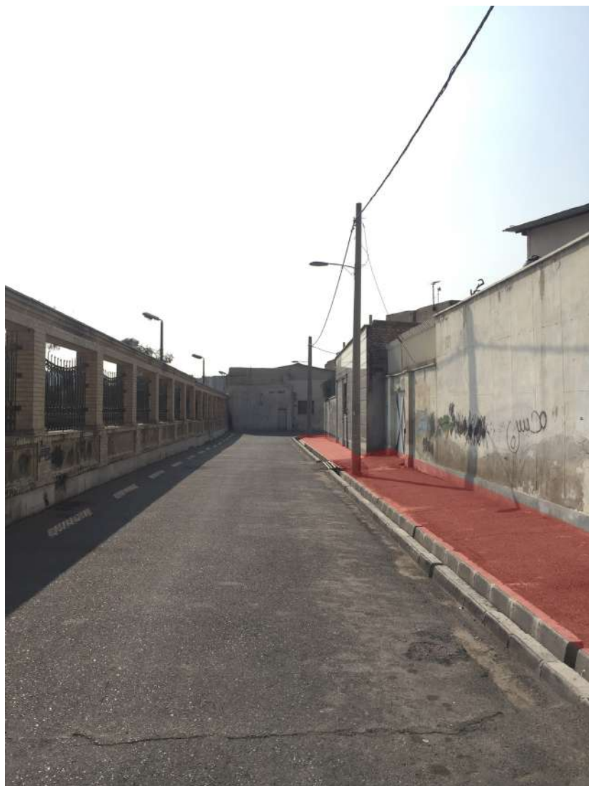
Fig.108: The sidewalk - North -West side of the cemetery, 2019
