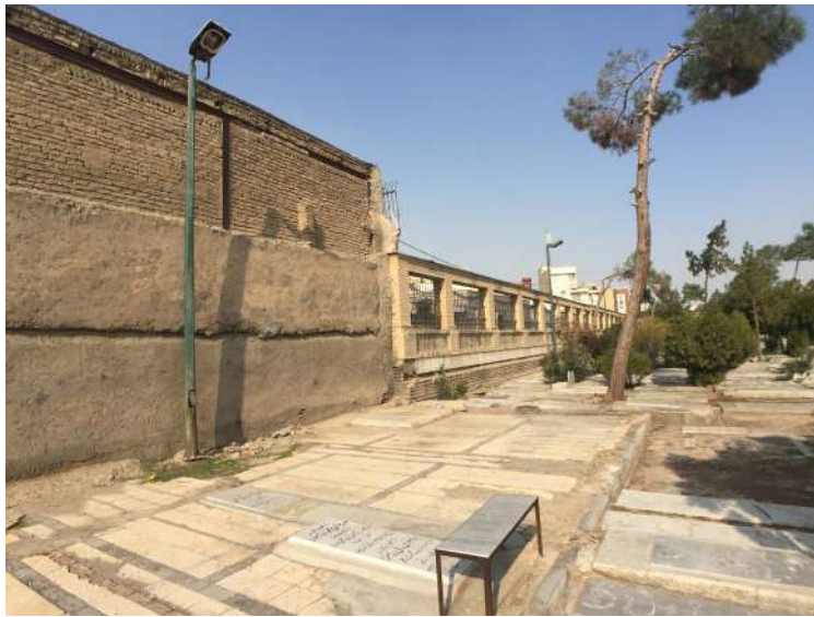
Fig.104: Low quality lighting system , 2020
