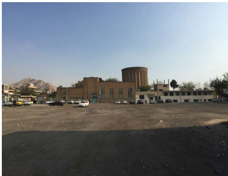
Fig.79: Empty space in the neighbourhood area without any function mostly use as a parking area, 2019
