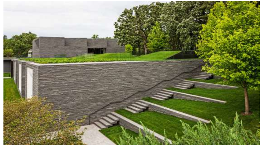
Fig.159: Stone scaled stairs faded into the slope and A green roof planted above the lower garden level
