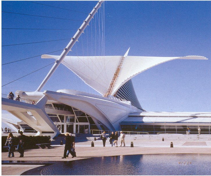
Fig.27. Milwaukee Art Museum, Wisconsin USA, 1994–2001, Santiago Calatrava.
