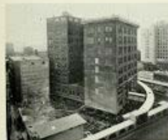
FIGURE 8. Two days later on October 30 shows one-third of the turn completed.
