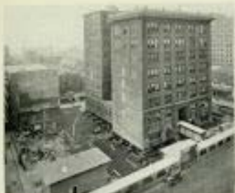
FIGURE 4. As the building appeared on October 14 ready for the move to start.
