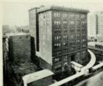
FIGURE 6. October 25 showing curved walk in place. The building turn has been started.
