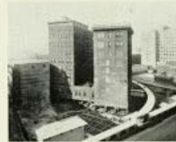
FIGURE 9. On November 1 the structure had moved around to the half-way point.
