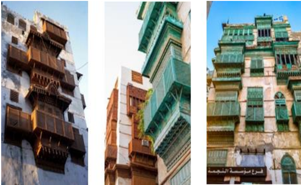
Figure 1.18. Examples of Jeddah's old buildings showing the wooden extruded windows on the facades with different colors (from different Sources).
