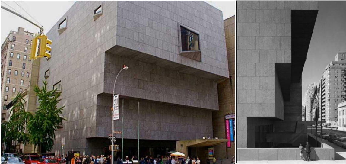
Figure 5.41. Designed by Marcel Breuer, Whitney Museum of American Art, New York, 1966. The overhanging facade of the building protects pedestrians from solar radiation. (Source: Photographer Ezra Stoller)
