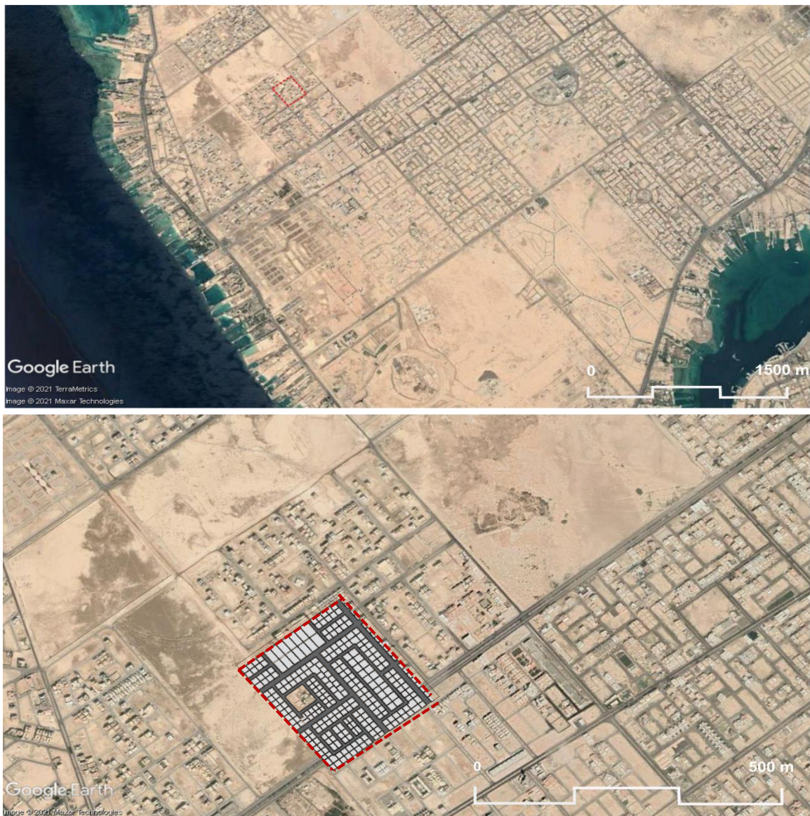
Figure 2.19. The case study Obhur AlShamalyah Low-rise buildings layout Case A (Source: Google Earth).
