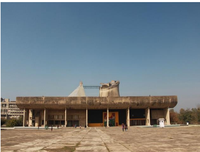
Figure 5.40. Designed by Le Corbusier, Palace of Assembly, Chandigarh, India, 1951. The designed shading element protecting the different entrances of the building: people can move from one access to another under the overhanging facade.
