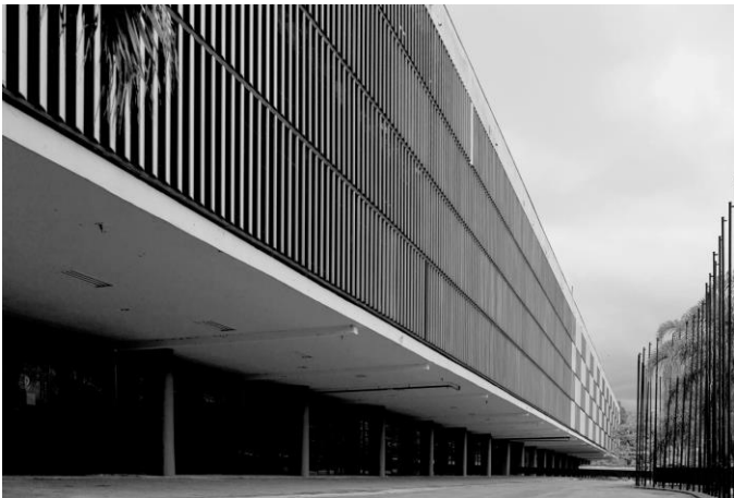
Figure 5.39. Designed by Oscar Niemeyer and Hélio Uchôa, Biennale Pavilion, São Paulo, Brasil, 1957. The overhanging facade clearly shows the shading view factor effect.
