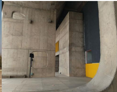
Figure 5.40. Designed by Le Corbusier, Palace of Assembly, Chandigarh, India, 1951. The designed shading element protecting the different entrances of the building: people can move from one access to another under the overhanging facade.
