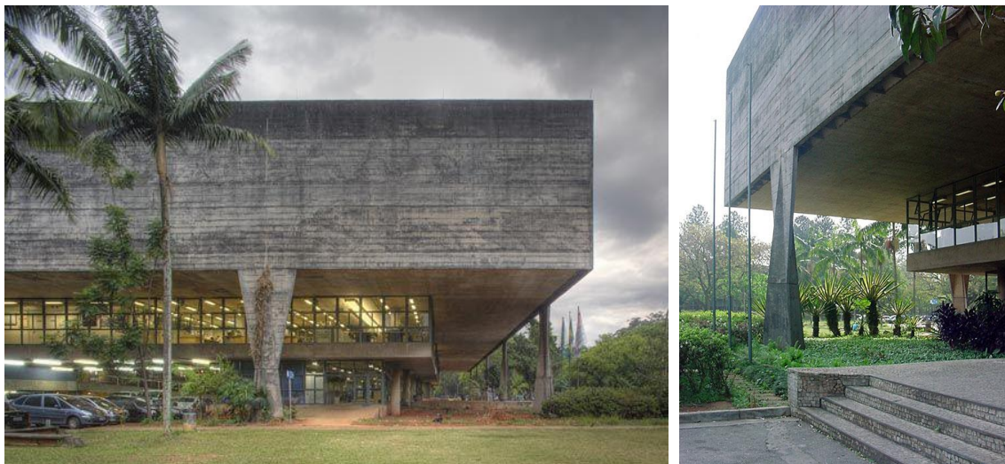
Figure 5.43. Designed by Carlos Cascaldi, College of Architecture and Urbanism, Sao Paulo, Brazil, 1961. A massive overhanging facade protects the entrance of the building.
