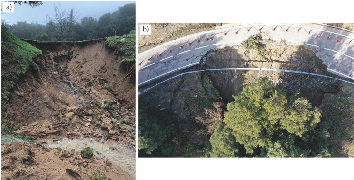
Figure 23. Examples of landslides triggered by the Gloria storm in the Montseny area. a) Rotational slide in a colluvium slope (photo courtesy of Clàudia Abancó). b) Rotational slide that affected a road embankment and parts of natural slopes (photo courtesy of Roger Ruiz)
