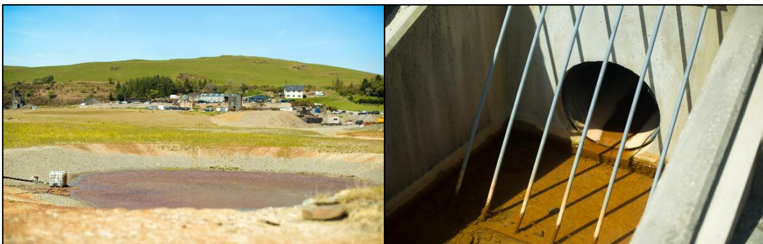
Figure 1.7: Frongoch (UK) abandoned metal mine impoundment and the channelling of the effluent release to the river.
