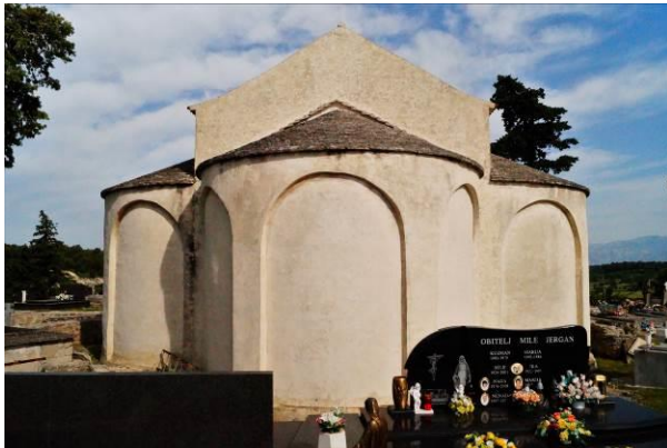
Fig. 79. Pridraga, Church of St Martin. View of the eastern apses
