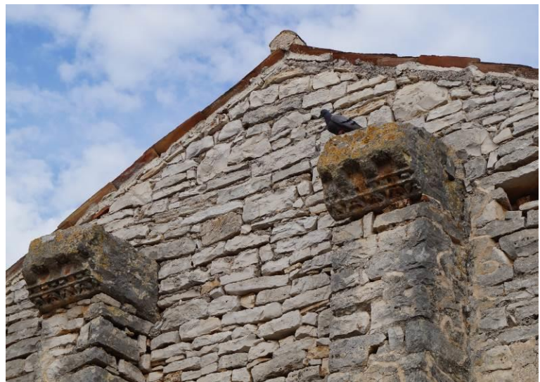
Fig. 47. Protruding structures of the western facade
