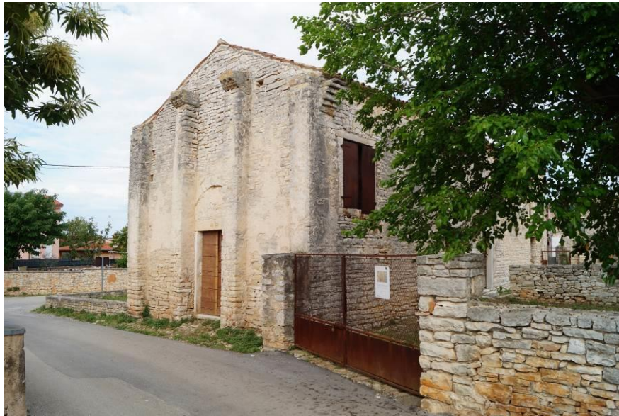
Fig. 45. Peroj, Church of St Stephen, western facade
