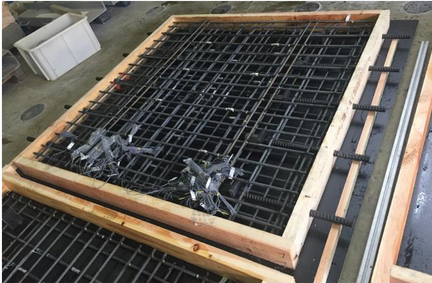
Figure 4.7: Position of post-tensioning bars inside the slab.
