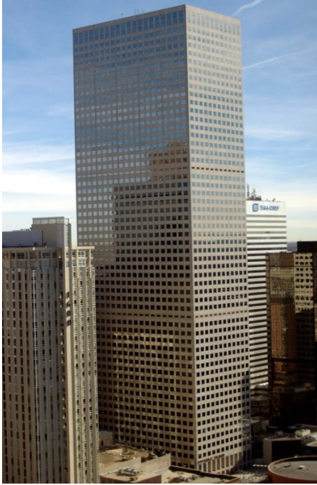
i) Republic Plaza Office Building Building Reference: Post-1980 Construction Year Built: 1984 – Renovated in 2016 Building Height: 56 Stories Façade Materials: Sardinian granite, Windows are flush-mounted with the aluminum grid
