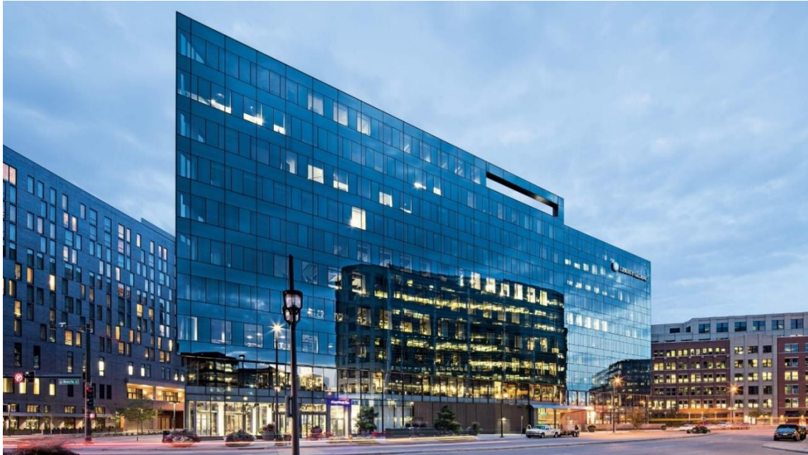
Figure 4.26: The Triangle Building office space, Denver, Colorado.
