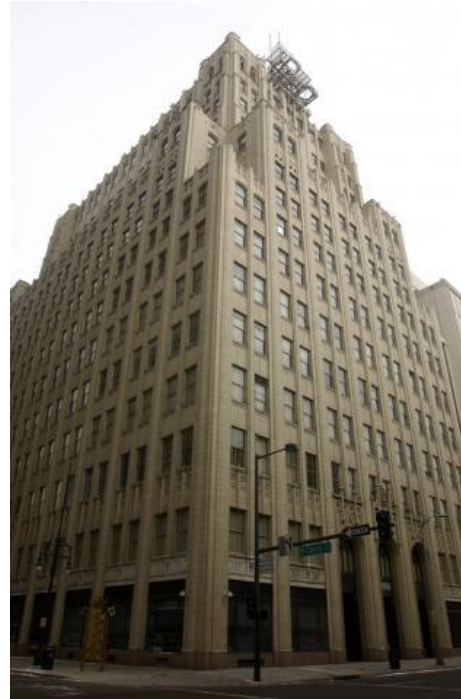
b) AT&T Office Building Building Reference: Pre-1980 Construction Year Built: 1929 Building Height: 24 Stories Façade Materials: Terracotta tiles, Granite, Steel, Glass
