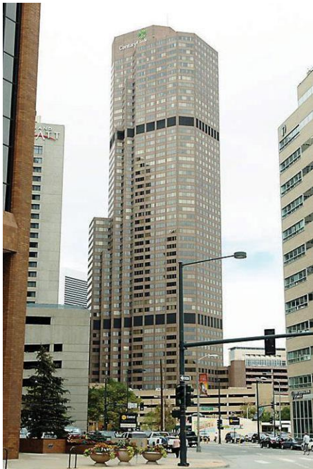
g) 1801 California Office Building Building Reference: Post-1980 Construction Year Built: 1983 Building Height: 53 Stories Façade Materials: Brown precast concrete, Curtain walling
