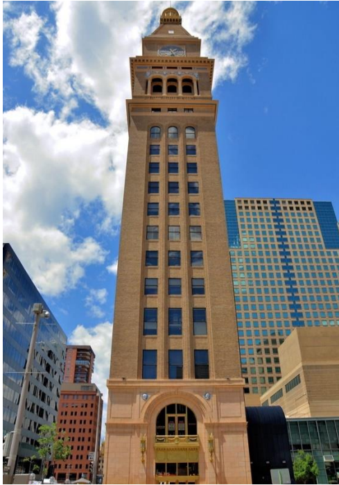
a) Daniels & Fisher Tower Office Building Building Reference: Pre-1980 Construction Year Built: 1910 – Renovated in 2006 Building Height: 20 Stories Façade Materials: Brickwork, Metalwork, Terracotta tiles, Glass
