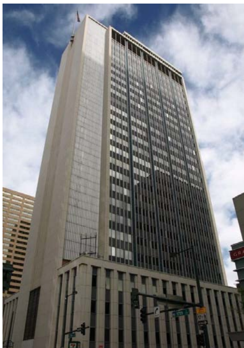
c) 621 17th Street Office Building Building Reference: Pre-1980 Construction Year Built: 1957 Building Height: 28 Stories Façade Materials: Stone, Glass
