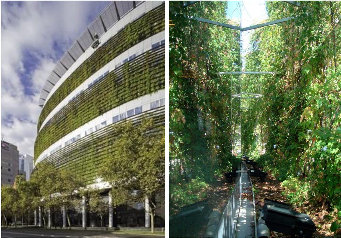
Figure 2.16: Consorcio Santiago Building, Chile.
