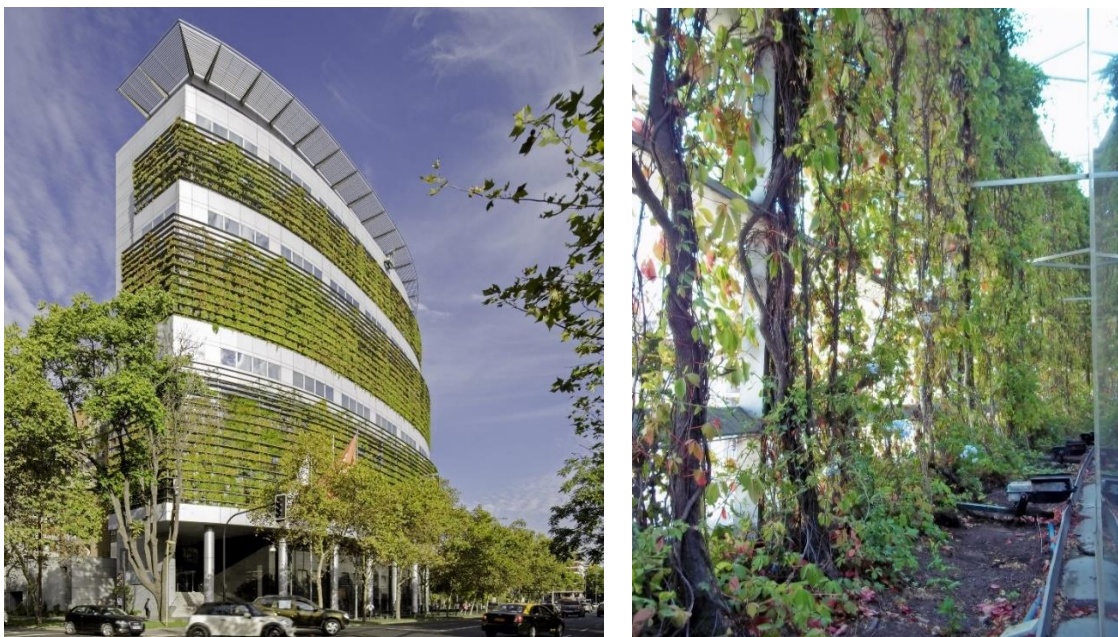
Figure 2.22: The 43% west façade greenery coverage of Consorcio project in Santiago, reduces solar gain by 60%, and the structure of green façade of Consorcio project.
