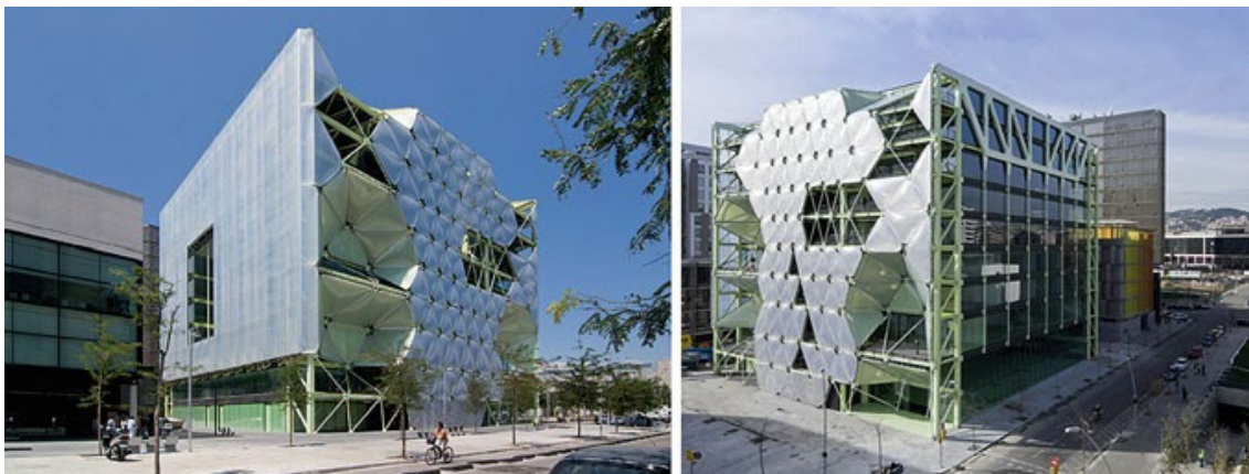
Fig. 4.1 – Media-TIC Building (authors: José Miguel Hernandez, Iwan Baan) 153
