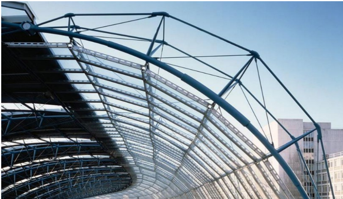
Fig. 4.6 - Waterloo International Terminal showing its glass panels that mimics a pangolin's scales (author: transformKC) 181
