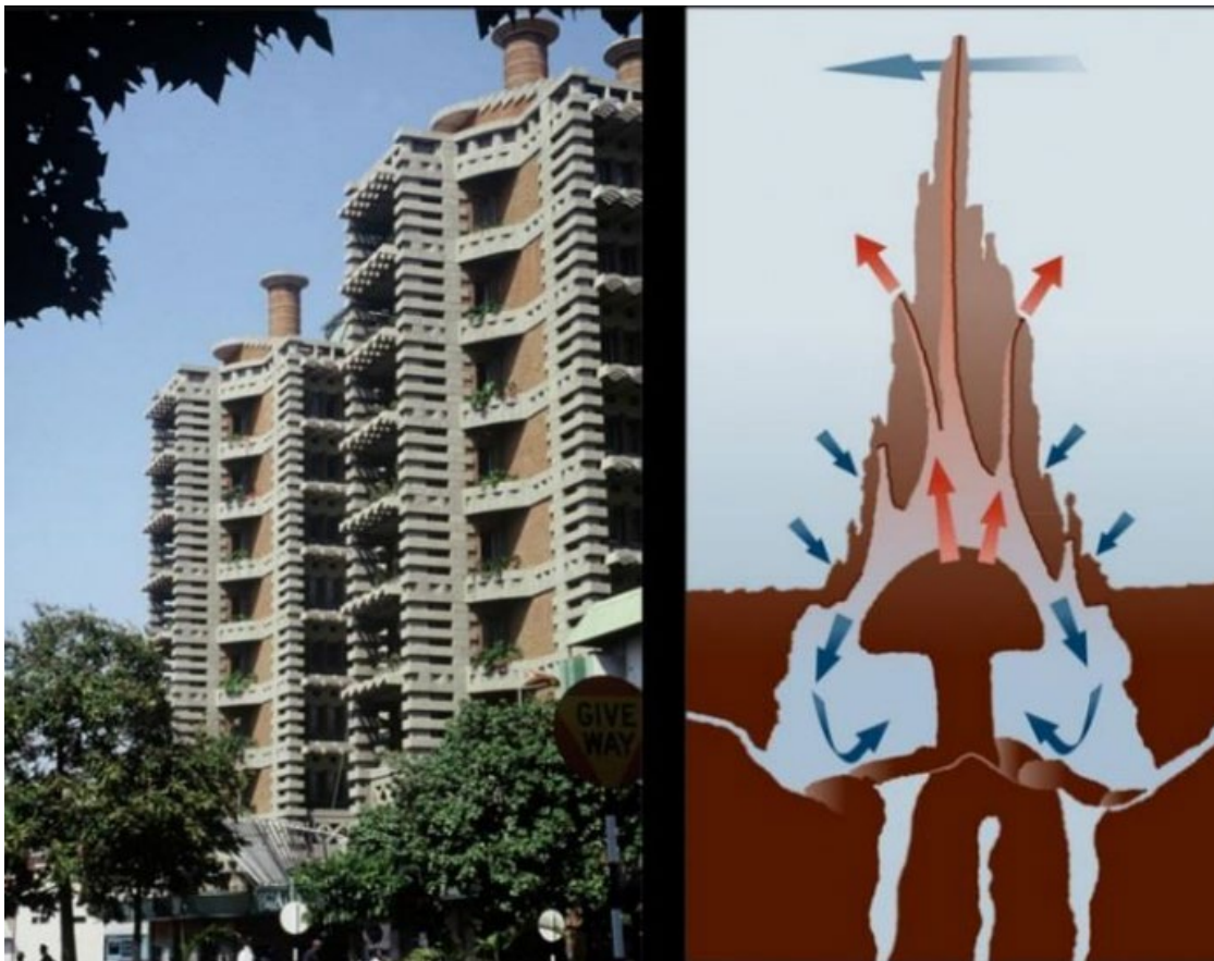
Fig. 4.7 - biomimicry application of a termite mound to employ a natural ventilation system in Eastgate Center (authors: David Brazier, Daniel Gallant, Mick Pearce) 183
