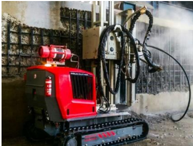
Figura 3-13 (a) Robot demoliendo (highimpactsolutions.com.au)
