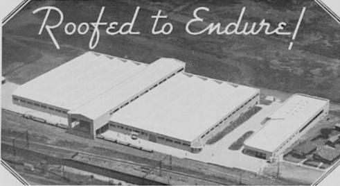
Approx. 112,500 sq. ft. of "FIBROLITE" Super-Six Corrugated Sheets were used for roofing, and 9,800 sq. ft. for walling, these large Works and Office buildings for Messrs. H. V. McKay Massey Harris Pty. Ltd., Concord, Sydney.
