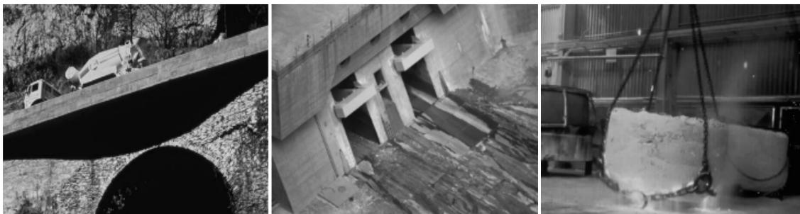
**Figure 2.2.** Typical applications of CAC concrete: 1. Bridge widening, rapid hardening. 2. Dam flushing gate, abrasion resistance. 3. Foundry floor, abrasion and thermal shock resistance. (K. Scrivener, J. Newman, 2003).
