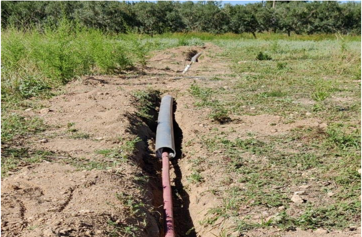
Fig. 47 Buried Horizontal dipole
