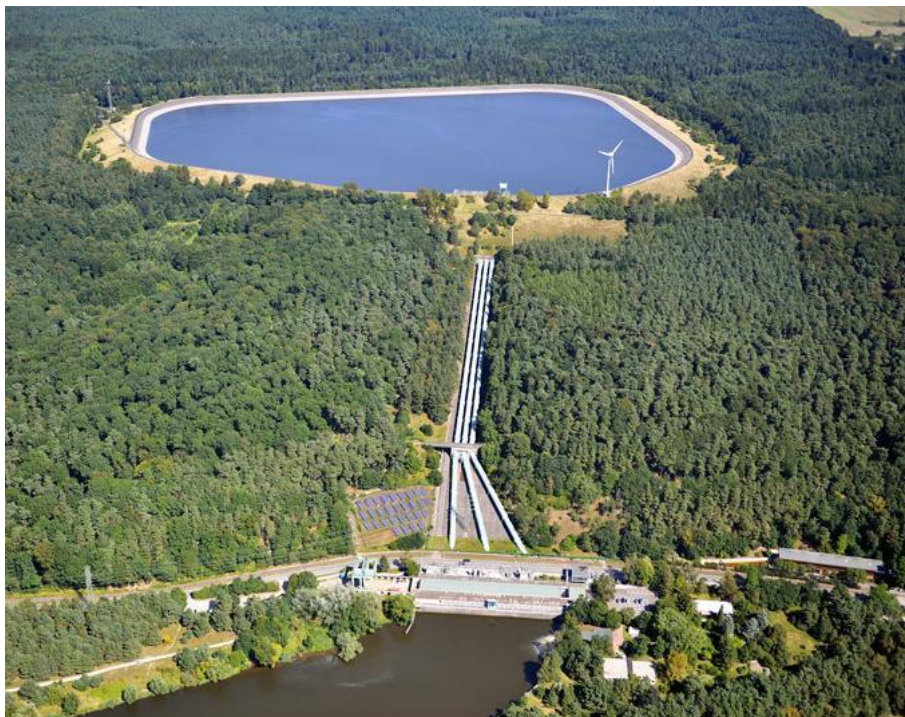
Figure J.1. The Geesthacht pumped hydro storage plant in Germany. Photo credit: Vattenfall AB
