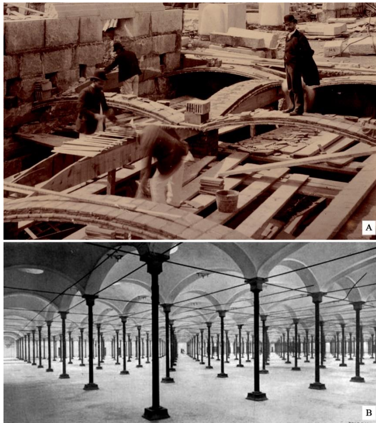
Fig. 1 Example of two buildings with timbrel vaults using thin clay tile. A) Guastavino standing on a timbrel arch with the timbrel vaults under construction [Photograph adapted from [25], distributed under a CC BY 2.0 license].
