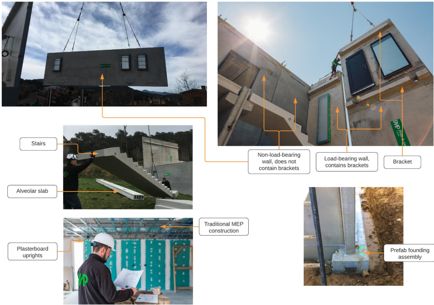
Figure 4-5. PMP construction process
