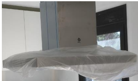
Figure 5-5. Sealing the kitchen fume hood
