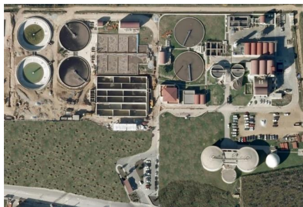
Figure 2.5 Aerial view of a Waste Water Treatment Plant
