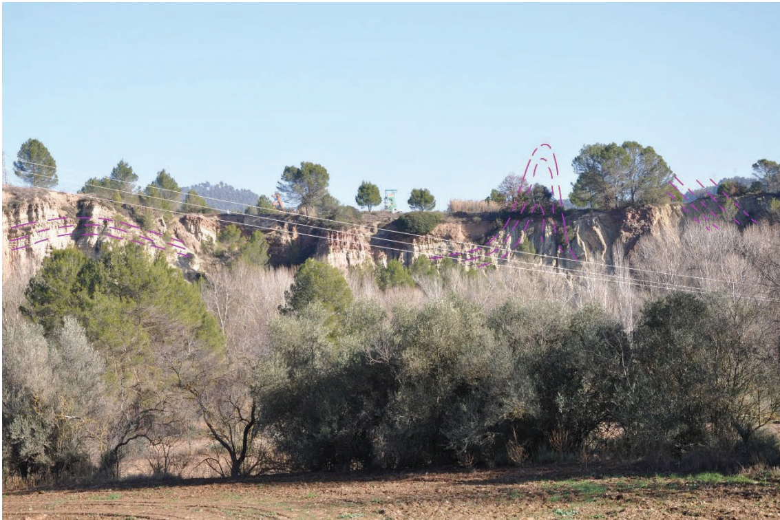
Figure 1.9 General view of the Sucova structure ( Adapted from Fàbrega et al., (2007)).
