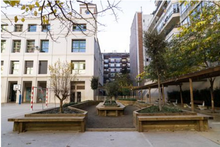
Figure 1 - A schoolyard transformed into a climate shelter in Barcelona. Interventions include a new garden with drought-tolerant trees and herbs, unsealed pavement, a gazebo with a vine, water points and seating arrangements. Source: Ajuntament de Barcelona
