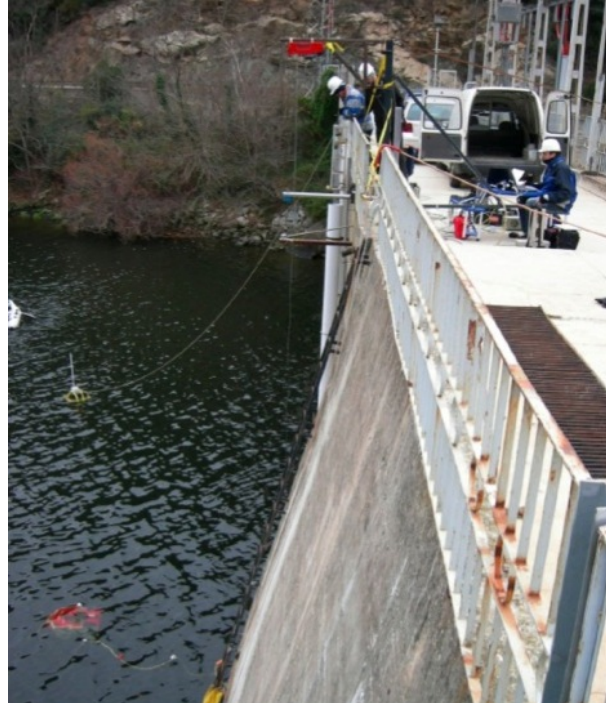
Figure 8.1: Dam inspection setup during the experiments carried out in Girona (Spain).
