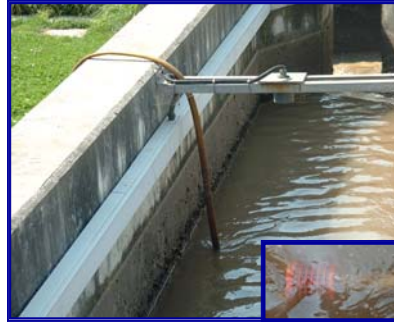
Figure 3.5. Picture from the WWTP where the wastewater was taken as an influent for the SBR pilot plant.
