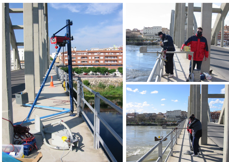
Figure 1. Portable cranes used for sediment transport sampling
